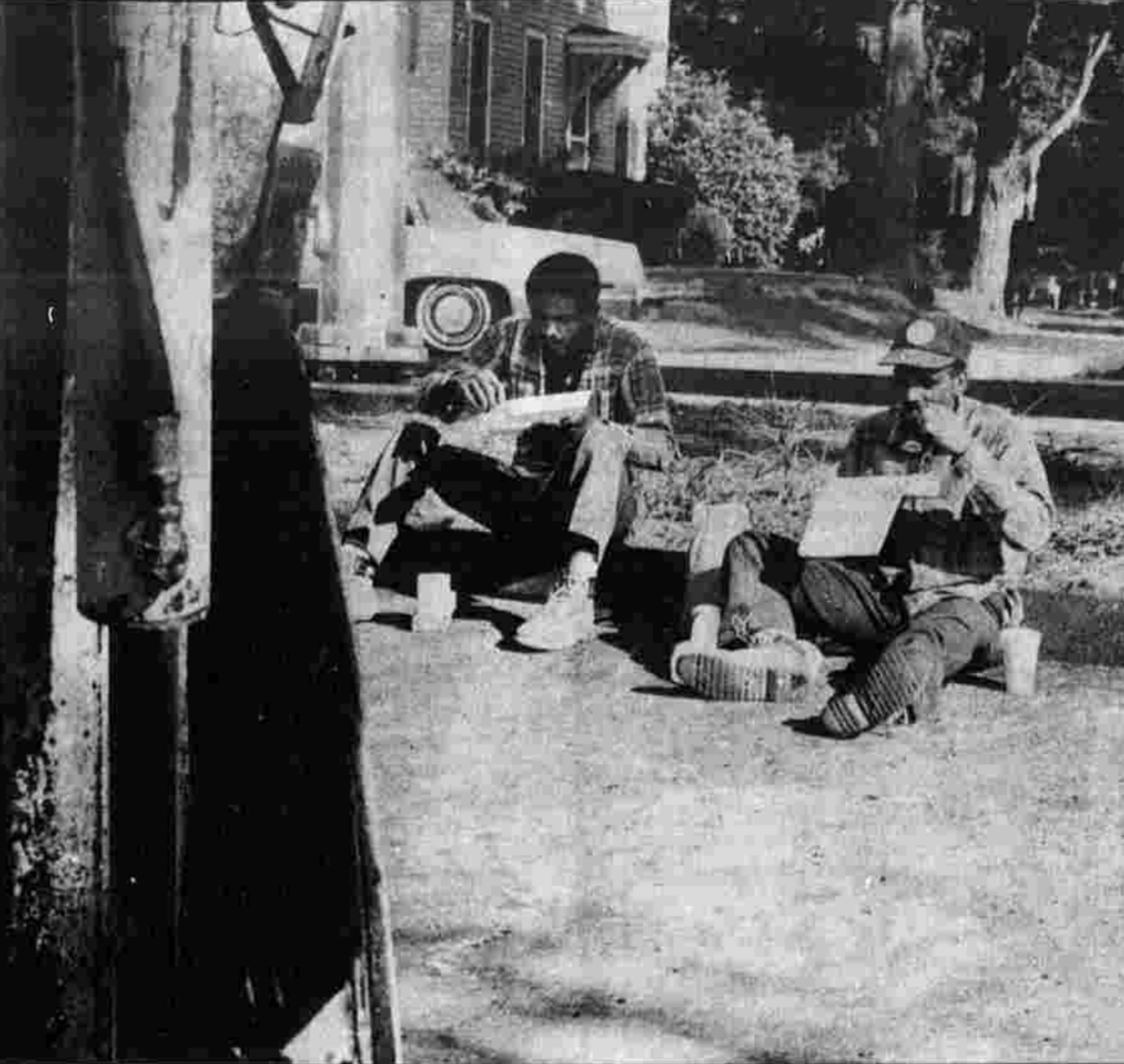
LUNCH BREAK — Concrete workers Remoaldo Cardoso, left, and Antonio de Pina, both of Norwalk, take a well-earned lunch break on Charter Oak St. in Manchester. The two men work for P.D.F. Construction Inc. of Waterford.
